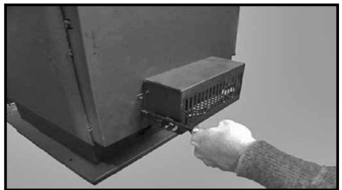
Figure 18: Installing the blower.
