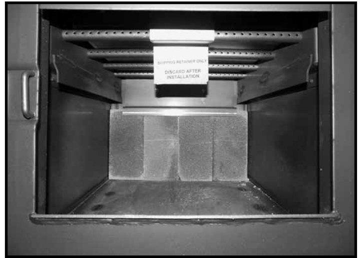
Figure 20: Bricks against rear wall.
