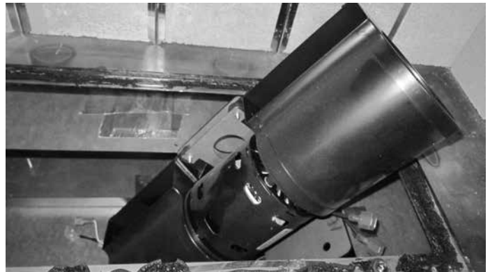
Figure 4.14 Remove Fan from Access Hole
