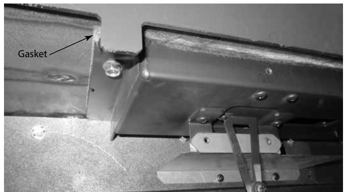
Figure 4.22 Install New Air Chamber
