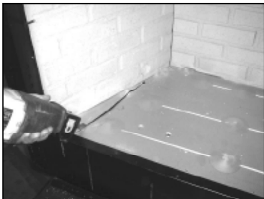
Figure 11.2. Using a saws-all, cut out the floor.
