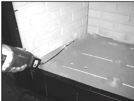
Figure 11.2. Using a saws-all, cut out the floor
