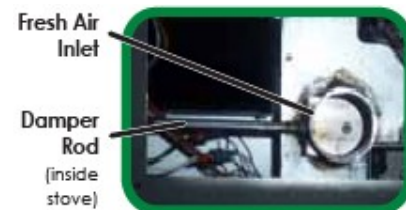
Damper Rod (normally located on rear side panel)
