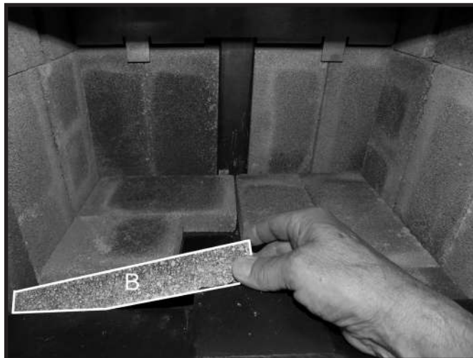
Figure 30: Final narrow brick in place.
