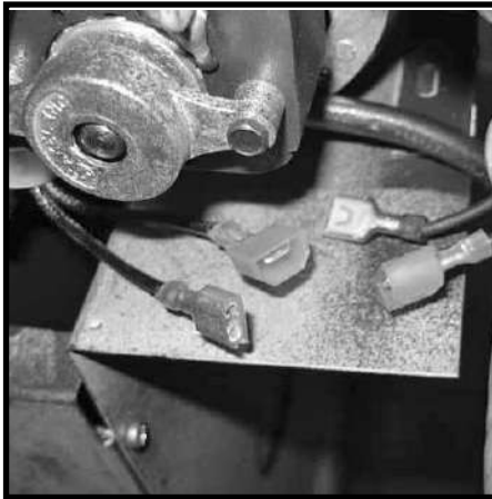
Figure 13: Disconnecting fan wires.
