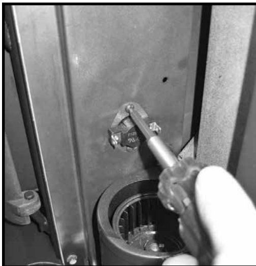
Figure 20: Removing thermal switch.
