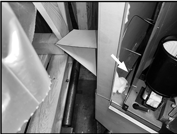
Figure 26: Rating label in place.
