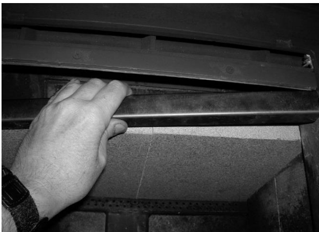
Figure 18 - Removing/Replacing the Baffle for Inspection
