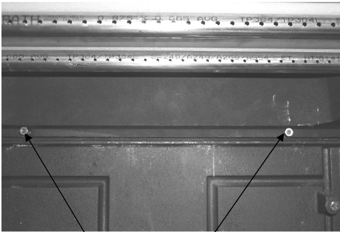
Loosen these socket head screws to allow baffle to come out of the firebox
