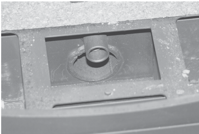
Figure 35: Remove ash from ignitor tube (underneath firepot)
