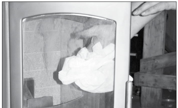
Figure 31: Wipe glass and inspect gasket
