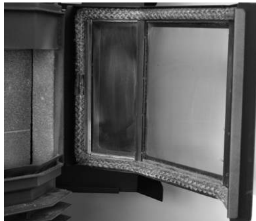
Figure 15: Wipe glass and inspect gasket
