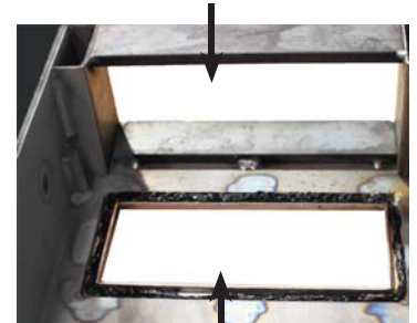
BYPASS DOOR OPENING
