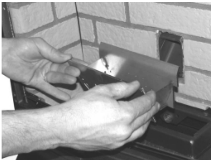
Lift the firepot out of the firebox.
