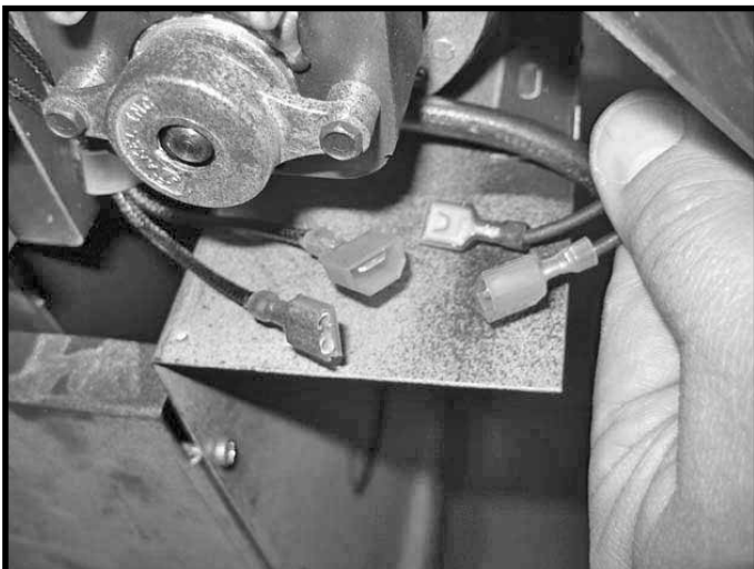
Figure 21: Disconnecting fan wires.
