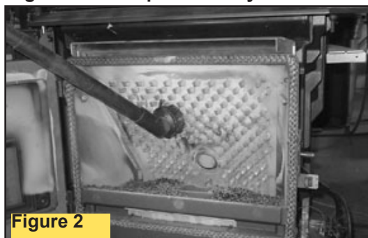
Figure 1 - Example of a dirty heat exchanger
