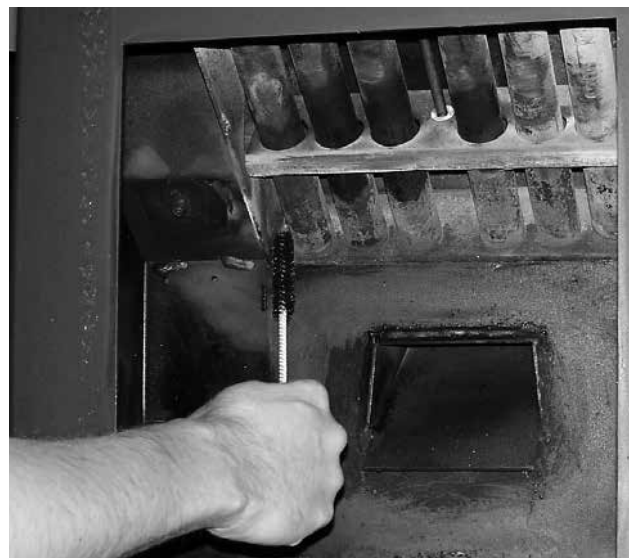
Figure 25 - Clean Behind Tube Scraper
