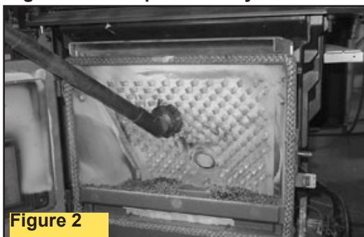
Figure 1 - Example of a dirty heat exchanger
