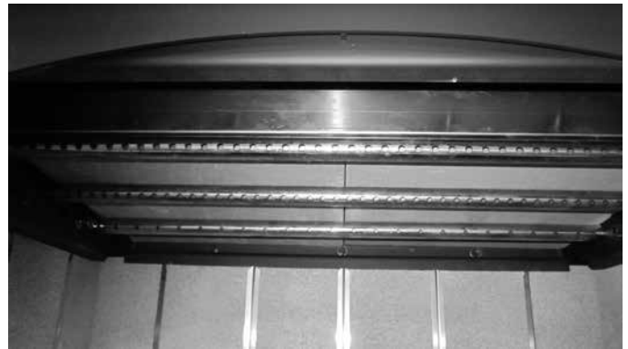
Figure 4.8 Reinstall Baffle Boards
